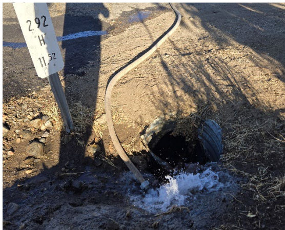
Flushing Culvert at Lake Rd./Banducci Rd.
