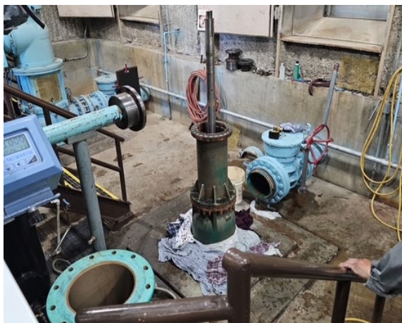
7-Stage Pump Replacement at PP1-E2
