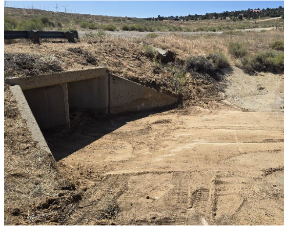
Cleaned Out Drainage Culvert
