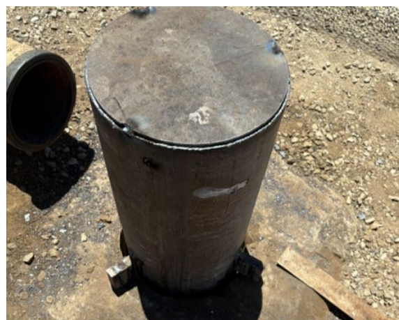
12-inch Steel Liner Installed at Nunes Well
