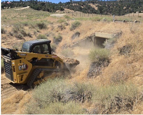
Drainage Culvert Clearing in Mountain Meadows
