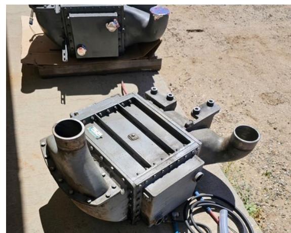
Intercooler Replacement at PP4
