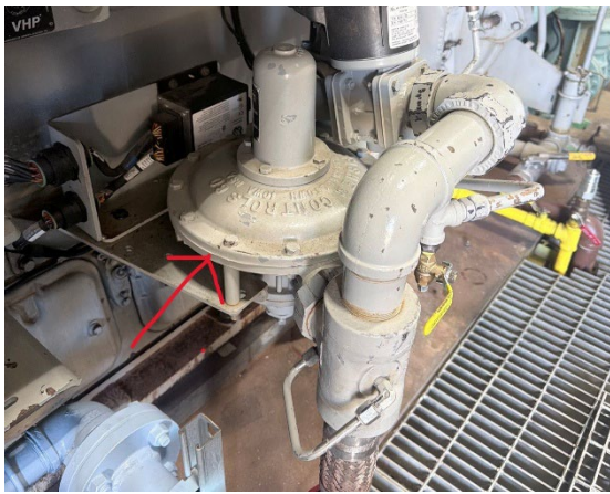
Gas Regulator Replacement at PP1
