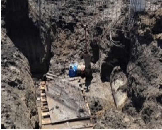
Mainline Turnout Repair in Cummings Valley
