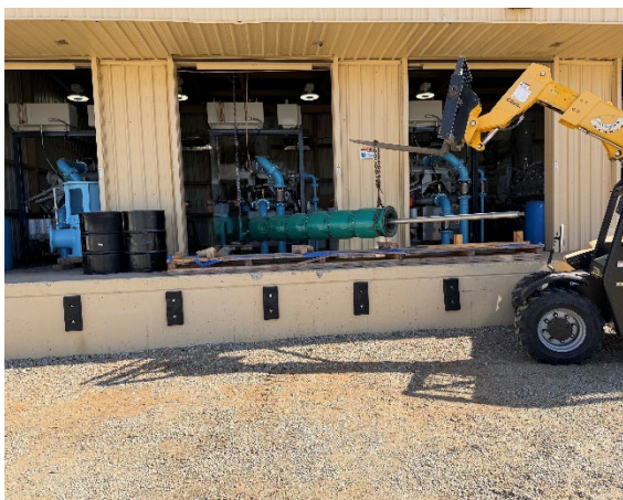
Reinstalling 7-Stage Pump at PP2-E1
