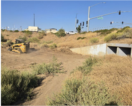
Cleaning Drainage Culvert at Teh. Blvd.
