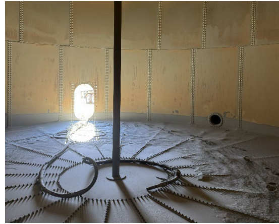
Oak Creek Tank Interior Coating Prep
