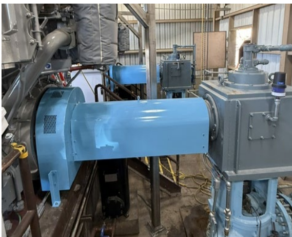
New Driveline Guards Installed at PP2
